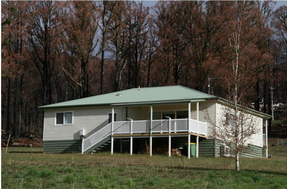
**Picture Captions:** Rowan intentionally constructed the house a respectable distance from vegetation and chose fire-retardant materials, including vinyl. He incorporated several energy efficiency principles such as good insulation and keeping the house airtight using double-glazed windows.
